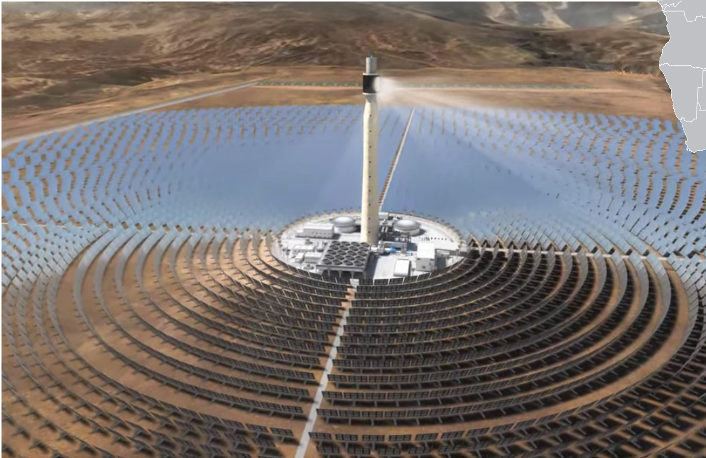
Ouarzazate Solar Power Station, also called Noor Power Station is a solar power complex and auxiliary diesel fuel system located in the Drâa-Tafilalet region in Morocco, 10 kilometres from Ouarzazate town, in Ghessat rural council area. At 510 MW, it is the world's largest concentrated solar power plant.
